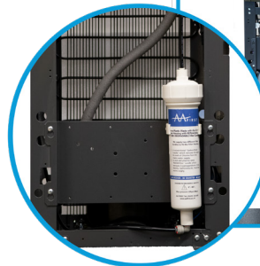
In a soft water area you only need a Carbon Filter to connect to the Boiler and the Chiller inlet
